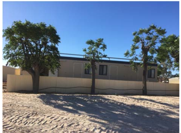
Accommodation unit at Innamincka ready for roof cover
